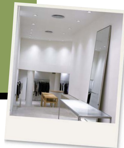
Ceiling Concealed Duct
